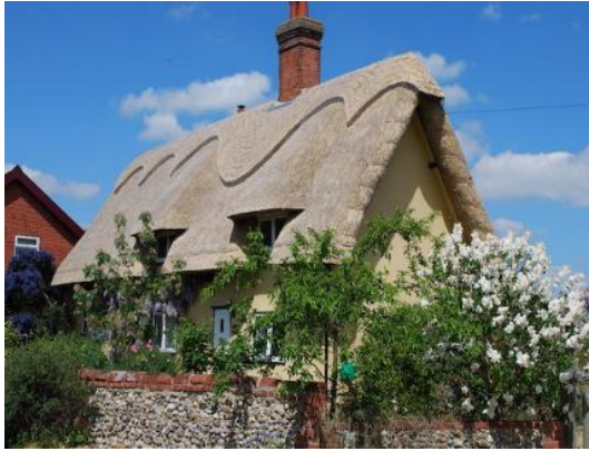
Chapel House, The Street
